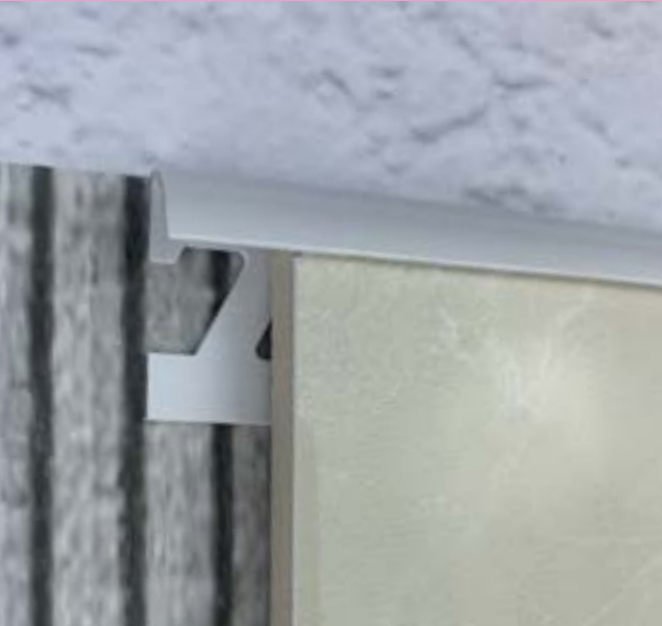
Chiusura perimetrale a muro/ Wall covering edging
